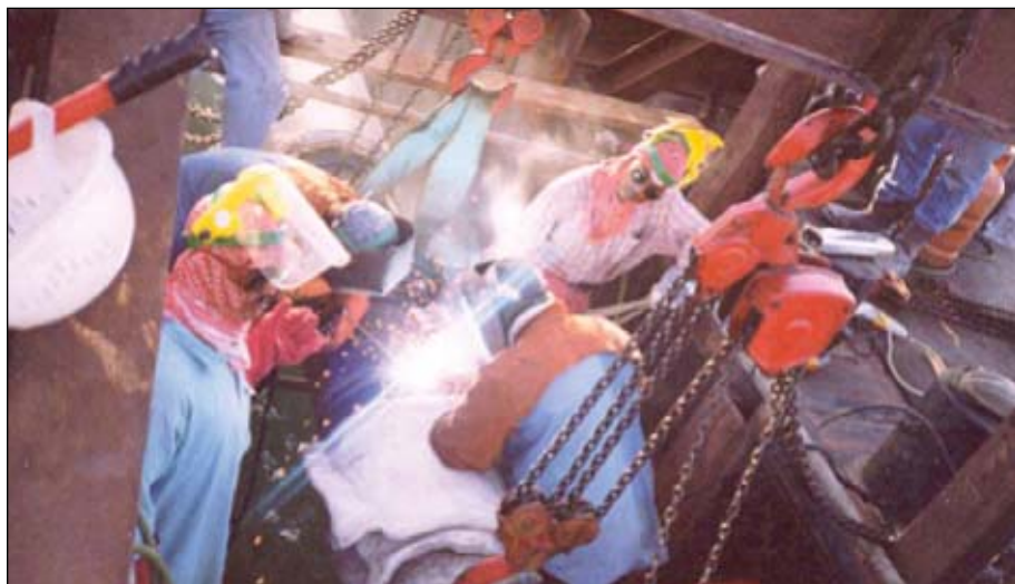
Offshore field tie-ins used welding on pontoons from which completed lengths were lowered (Fig. 8).
